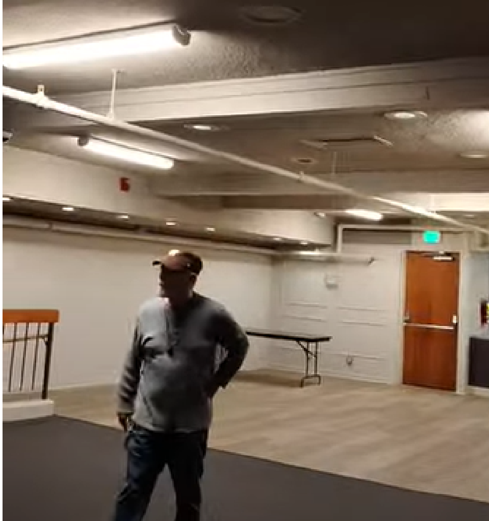
Figure 6: Same room from the opposite direction. One folding table. No resident chair setup for a meeting. Ceiling tiles and fixtures in place. The space is not set up as a usable community room.
