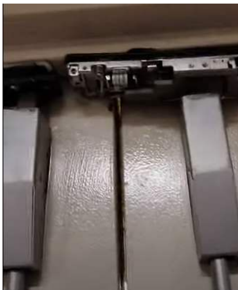
Door edge. Latch hardware separated. Strike not seated.
