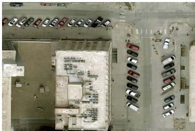
Aerial. Roof of the tower, condenser units, parking along the east side.
