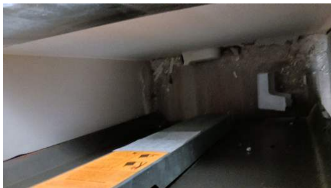
Gap beside an appliance. Debris on the floor. No cooking appliance in the opening.
