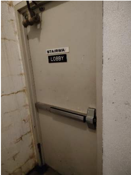
Door signed STAIRWAY / LOBBY. Panic bar on the occupied side. Hardware at the head. No padlock in this frame.
