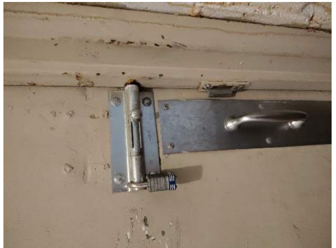
Slide bolt on the occupied side, held by a padlock.
