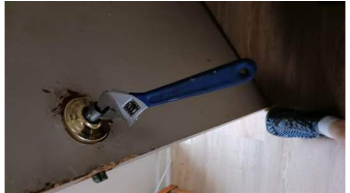
Unit door. Latch plate hanging. Makeshift knob of cord and a block.
