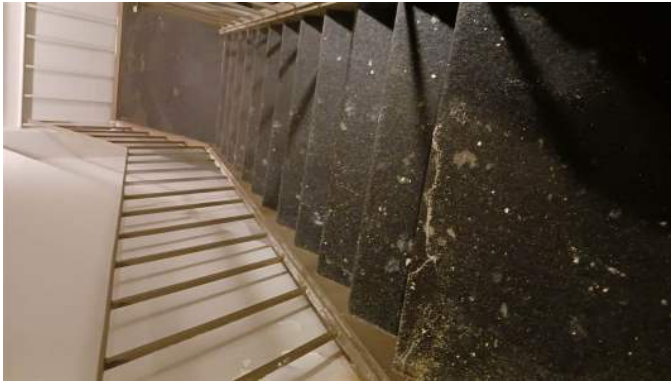
Stair side of a door. Chain and padlock through the panic hardware. Sign reads FIRE EXIT.
